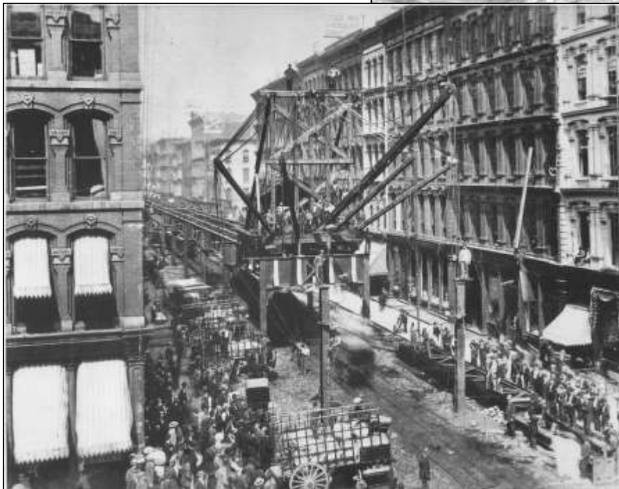
Construction of Chicago's transit system in 1895
